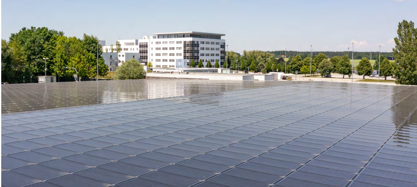
Photovoltaic system on the parking deck at the headquarters in Vilsbiburg.
